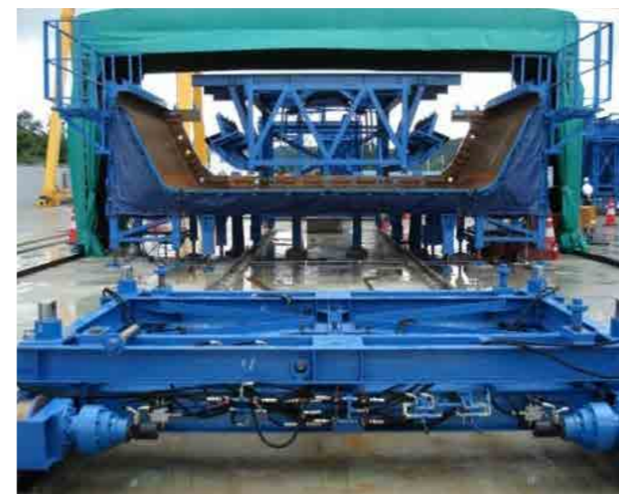
+ Uijeongbu LRT Project - Korea
