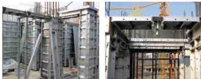
+3 Installation of beam and SC panels
