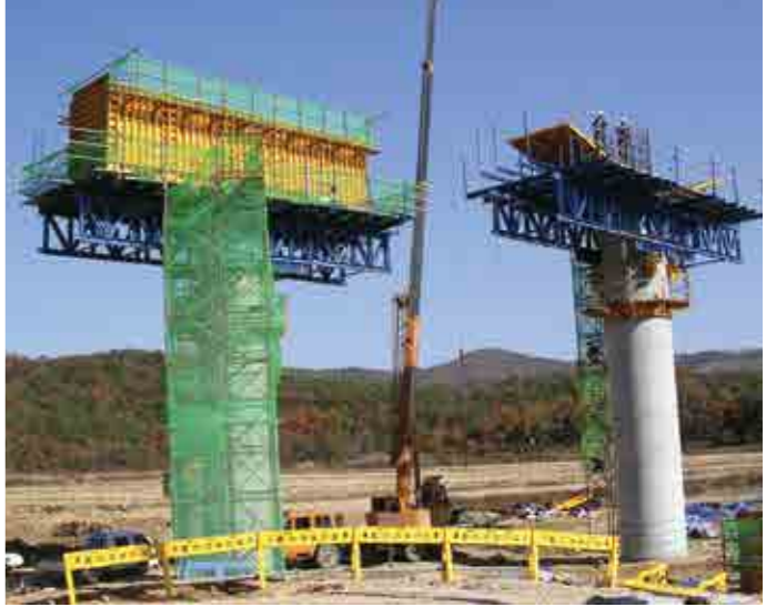
+ 1st section of Donghae Expressway - Korea
