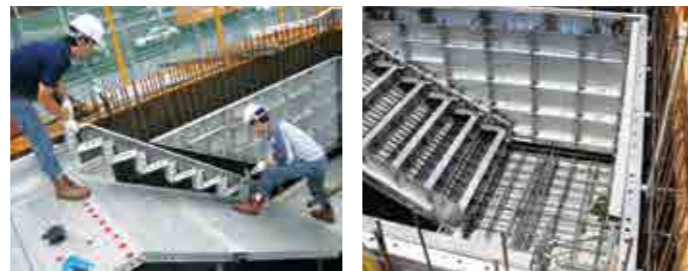
+4 Installation of staircase panels
