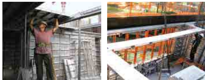
+5 Installation of slab panels
