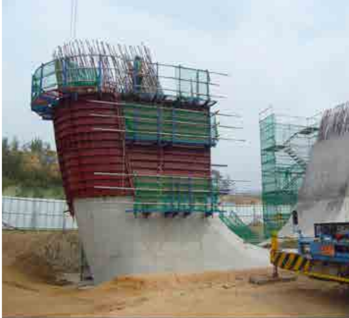
+ 4th Geumgang Bridge - Korea
