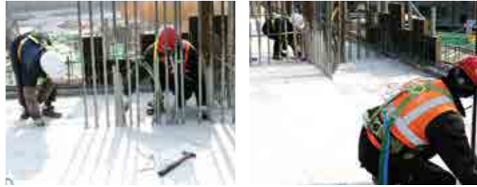
+1 Structural line and level check
