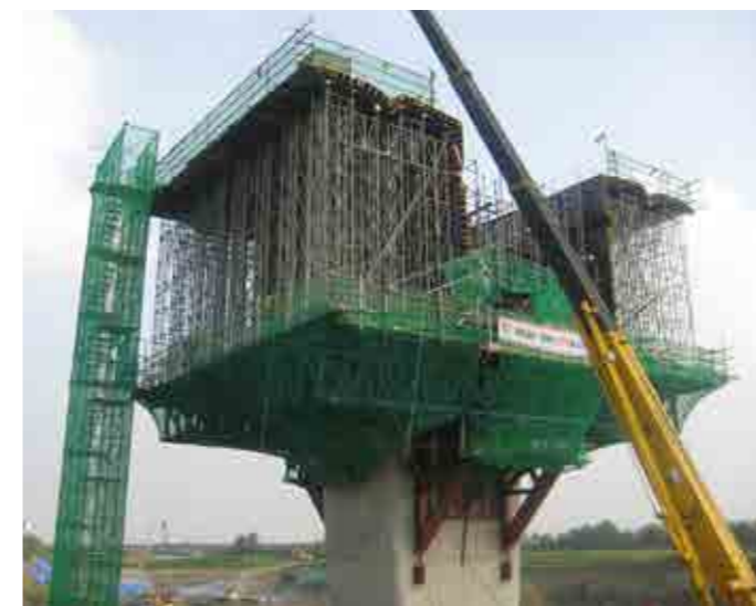
+ Soosong Bridge - Korea
