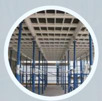
Considering the construction plan and repetitive use of formwork, Kumkang Kind's Slab system maximizes work efficiency by designing the formwork to be monolithic and fixed. Thus, it greatly increases the workers safety. By chaning the prop-head system to a drop-head system, safety against fallout of materials and noise problem has been reduced while dismantling has been considerably
