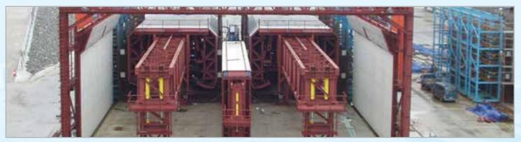
Kumkang Kinds Tunnel & Box Culvert system is widely used in general drains and passages to high-speed rail and immersed tunnels.
