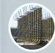
The timber-beam formwork is a classic system of the large-scale formwork which also called plywood formwork composed of the plywood, the timber beam and steel waling. This can be applied to any shape of structure and to a variety of jobsites such as foundation, walls, single-sided walls, retaining walls, piers and
